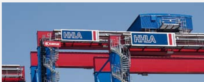
Automated cranes at work at HHLA Container Terminal Burchardkai
