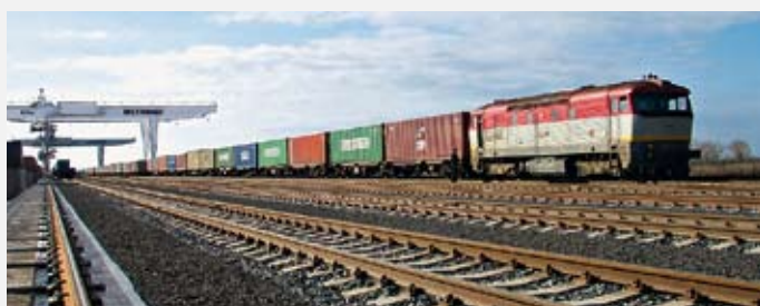
Handling station of the HHLA subsidiary Metrans in Dunajska Streda.
