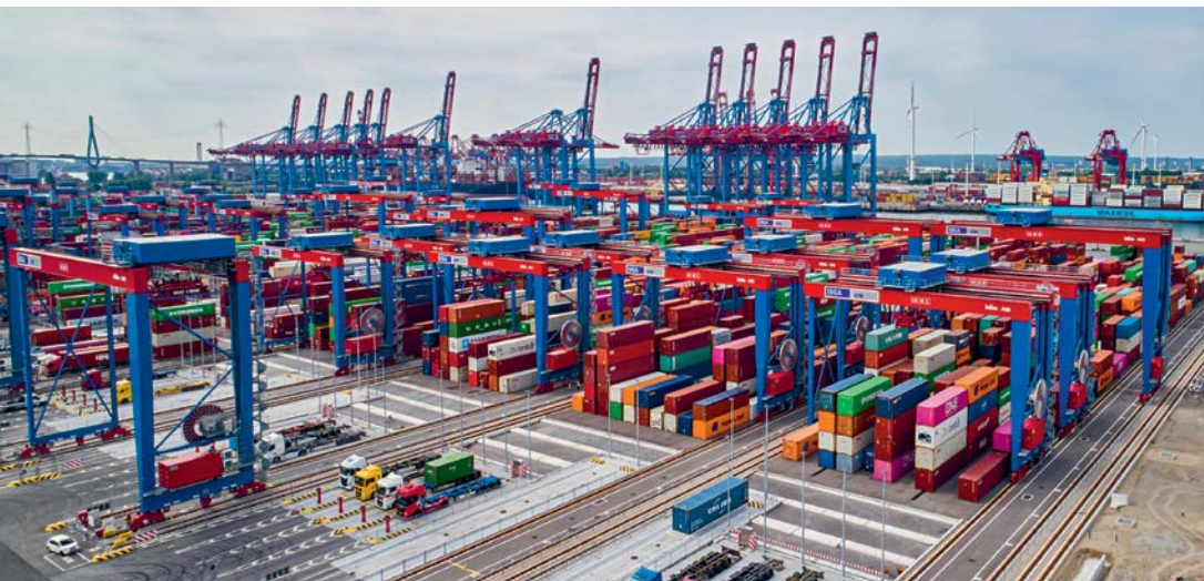
TIGHTLY PACKED A fully automated block storage system makes more efficient use of the space. It stacks the steel boxes higher and more densely so that more containers fit into the limited space at the Burchardkai terminal.
