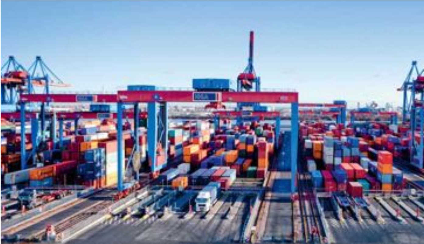
At the heart of Altenwerder's high-tech terminal: automated storage blocks with space for approximately 30,000 containers
