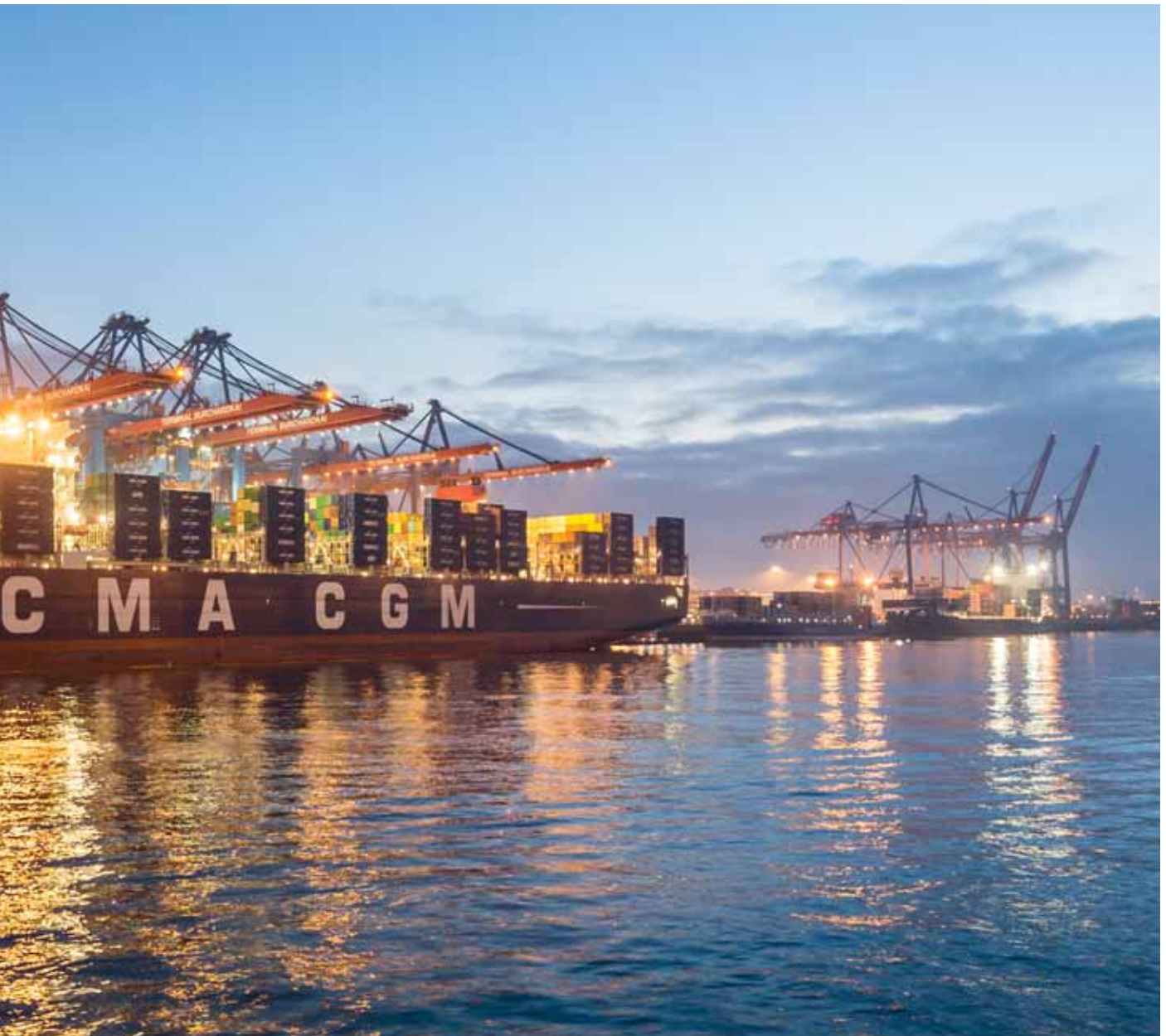
International hub: the world's largest container ship was handled at Burchardkai by seven gantry cranes simultaneously.
