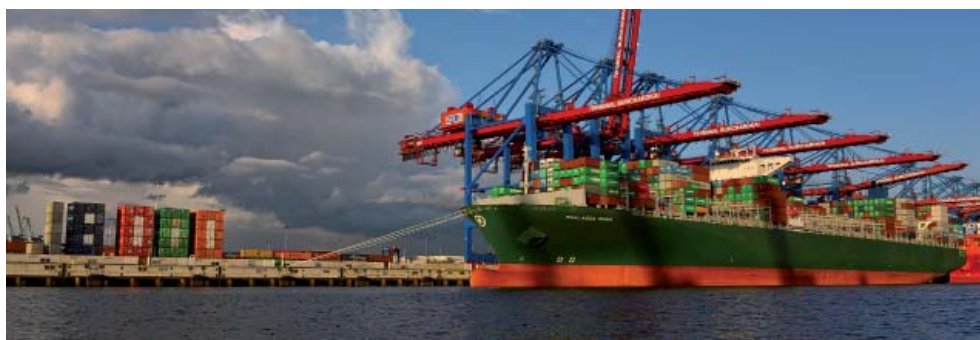
Further improvement in handling quality: the new mega-ship berth at the HHLA Container Terminal Burchardkai
