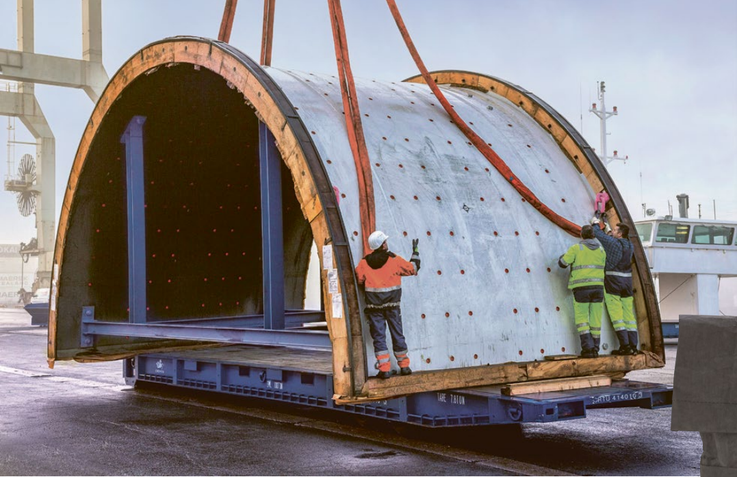
At the terminals, tension belts are used to secure heavy loads before they start their second life as backpack carriers.
